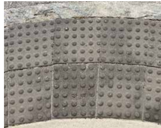
TRUNCATED DOMES Elizabeth City Truncated Dome, charcoal. When used in a radius, stones should be cut in appropriate sized wedges to follow the adjacent radius. Must be in compliance with ADA requirements for detectable warning surfaces.
